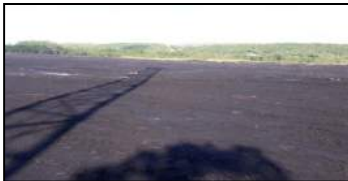
Gambar 4.1 Lantai ROM ( Base ROM )
